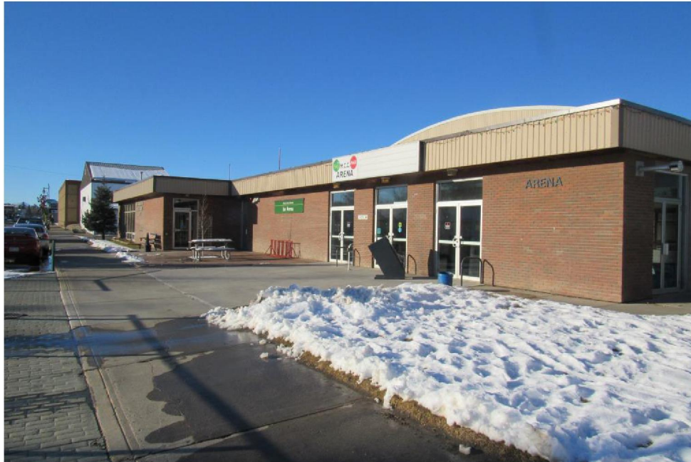
General view of the Site building.
