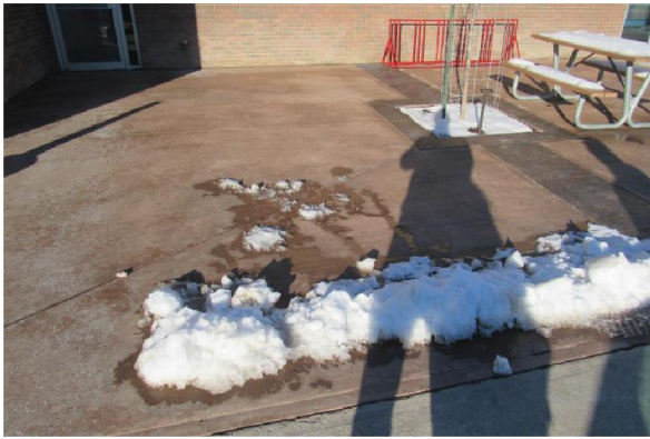
Photo #A3: Concrete pad walkway near front entrance.
