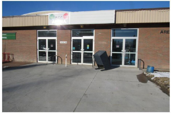
Photo #A10: Building main entrance.
