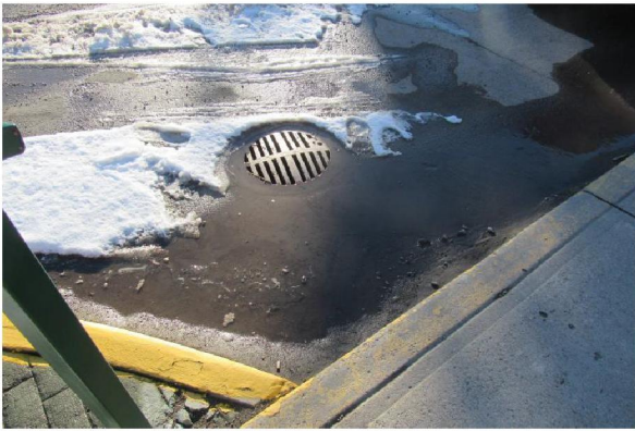
Photo #A9: Storm sewer in street near entry drive.
