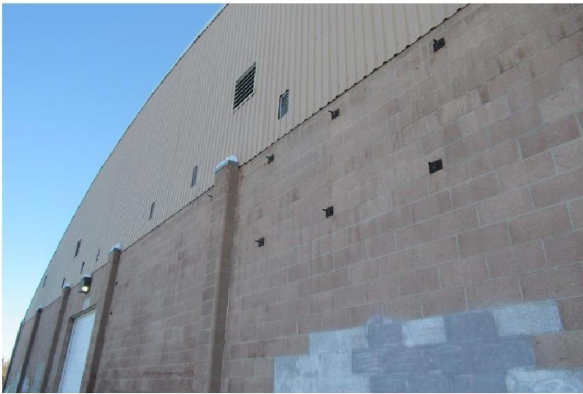
Photo #A5: Exterior cladding finishes.
