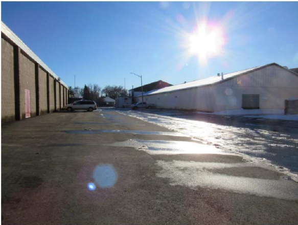
Photo #A1: Site parking lot.
