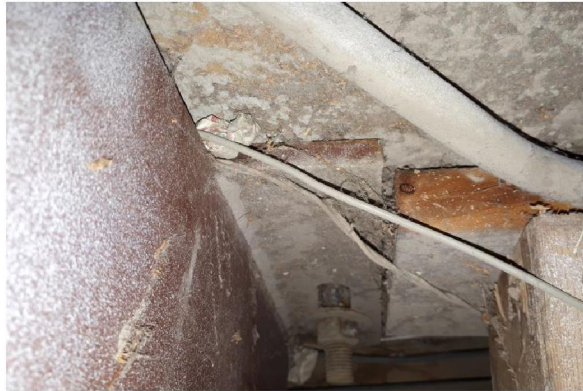
Photo #S7: Wood truss-concrete column connection.
