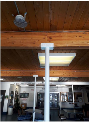
Photo #S1: Wood Beam-Steel Column in Lobby.
