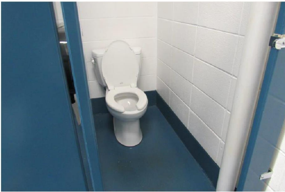
Photo #M3: Water closet fixture.
